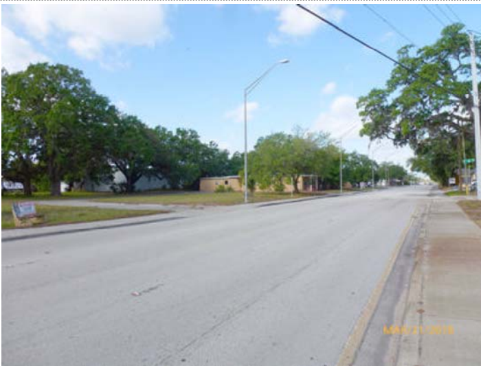
1. SR 64 E looking westerly
